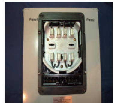
Retrofit Panel Adapter installed
