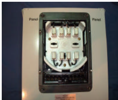
3. Retrofit Panel Adapter Installed
