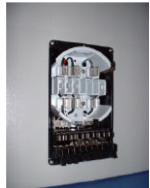
Retrofit Panel Adapter installed
