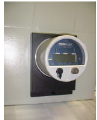
Retrofit Adapter installed with meter and cover
