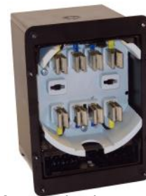
3. Retrofit Panel Adapter Installed
